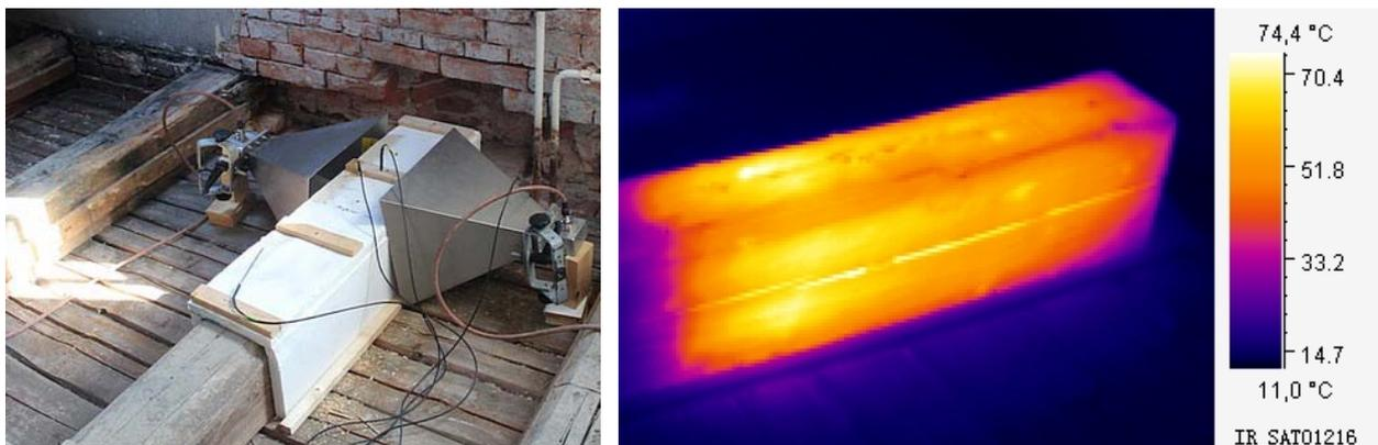
**Figure 3: Treatment of a ceiling beam, contaminated by dry rot (*Serpula lacrimans*), antennas on both sides, infrared recording were made shortly after completion of the treatment**
